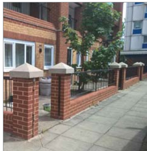
Example of Garden Wall to be Replicated
